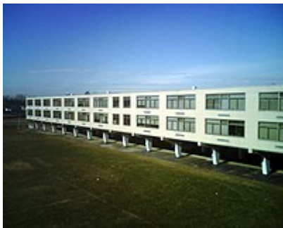
Rear view of Hicksville High School
